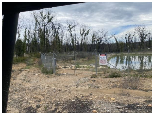
Plate 18: Basin water - signage not suitable for firefighting (4798).
