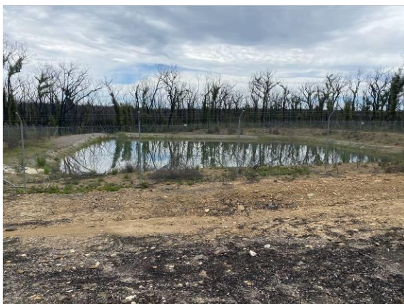
Plate 17: Basin - maintained clearance of tree vegetation (4796).
