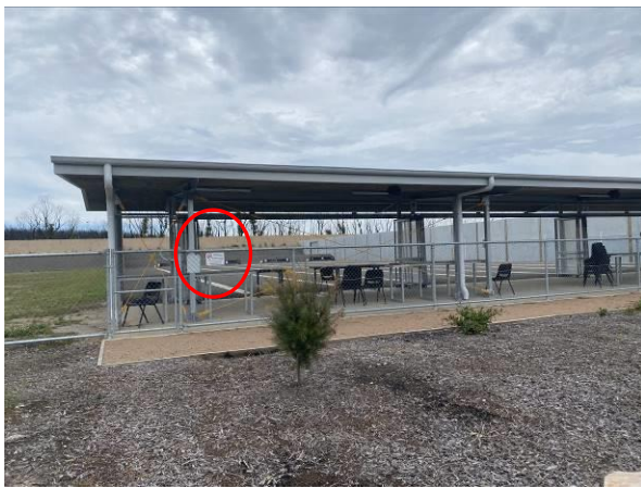
Plate 21: 50 m range - example of 'no smoking' signage (4814).
