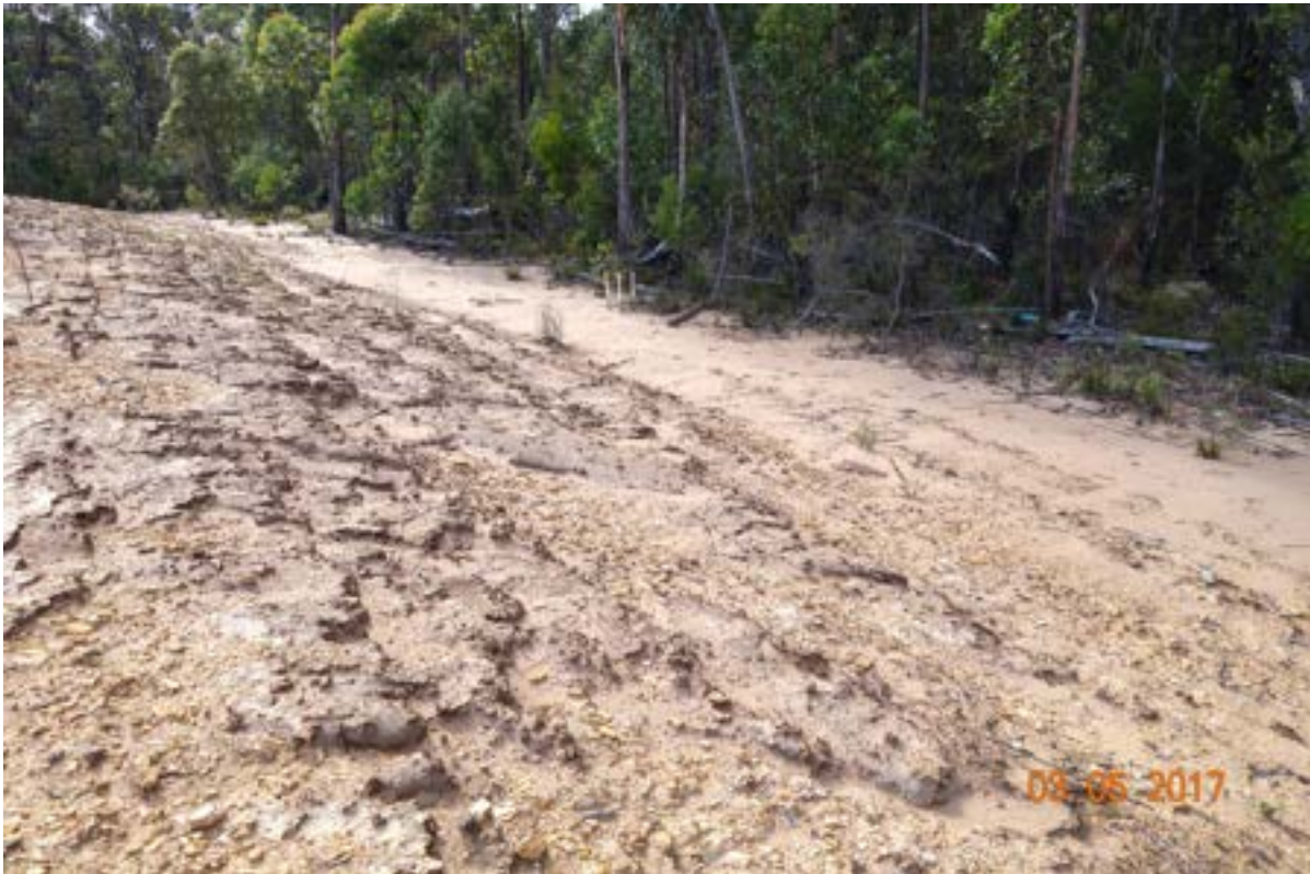
50m range: Outer slope of SE batter with erosion and deposition.
