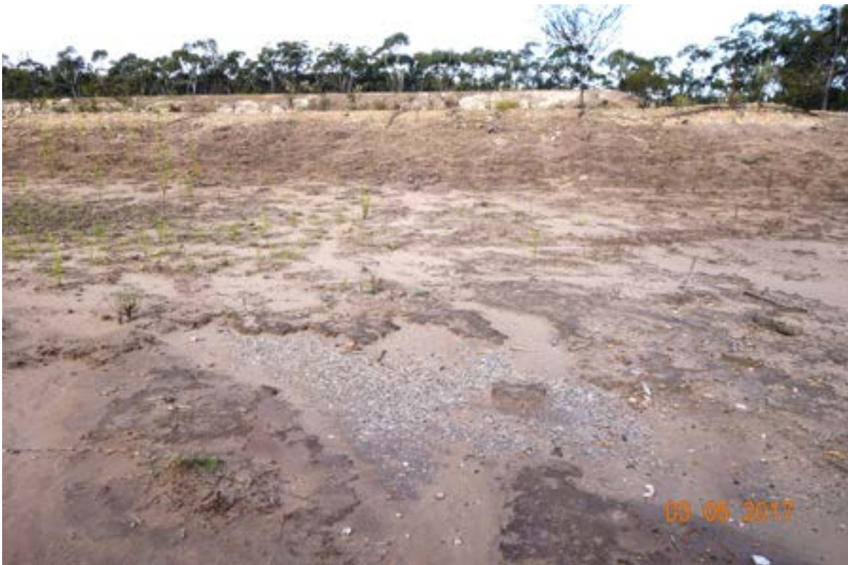
50m range: View across range to SW batter showing minimal revegetation, weeds and sheet erosion.
