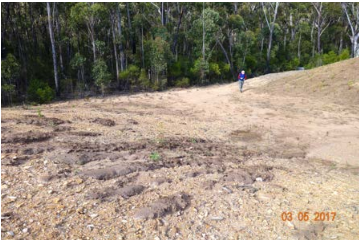
50m range: Junction of SE and SW batters with remnant topsoil, rilling and deposition.
