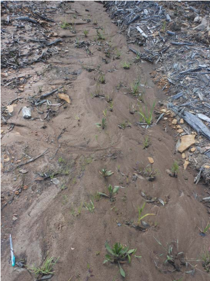
Photo 23 – Drainage ditch to sediment pond below Pistol Range
