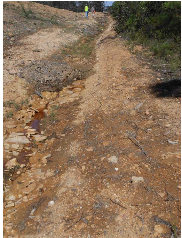
Photo 25 – Weeds in drainage ditch alongside sediment mound from 500m Range
