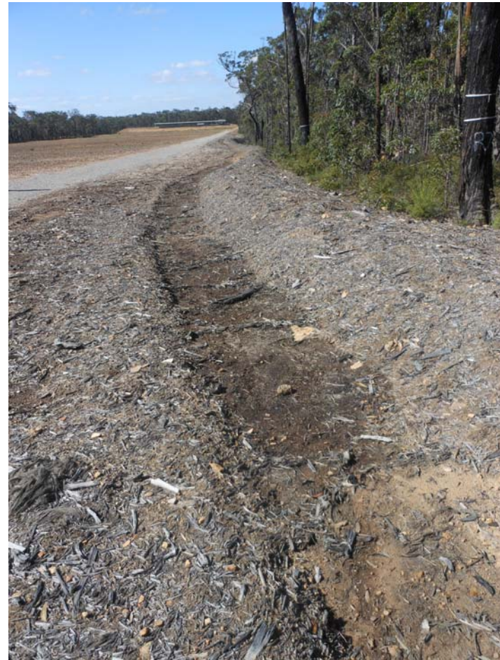
Photo 35 – Drainage ditch eastern side of 500m Range, weed free.
