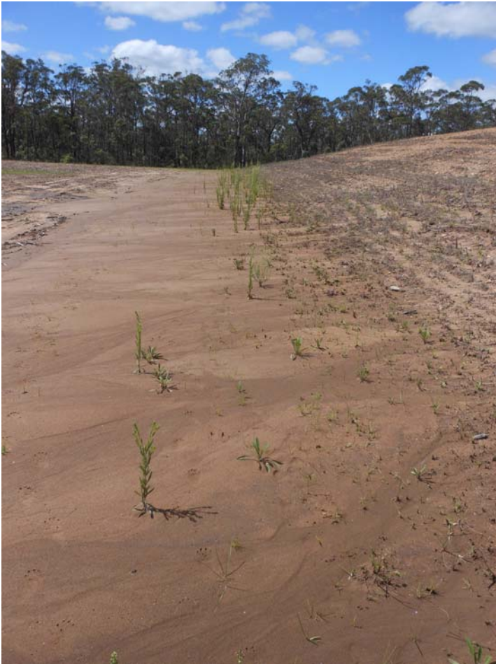
Photo 18 – Southern berm wall and base, less weeds
