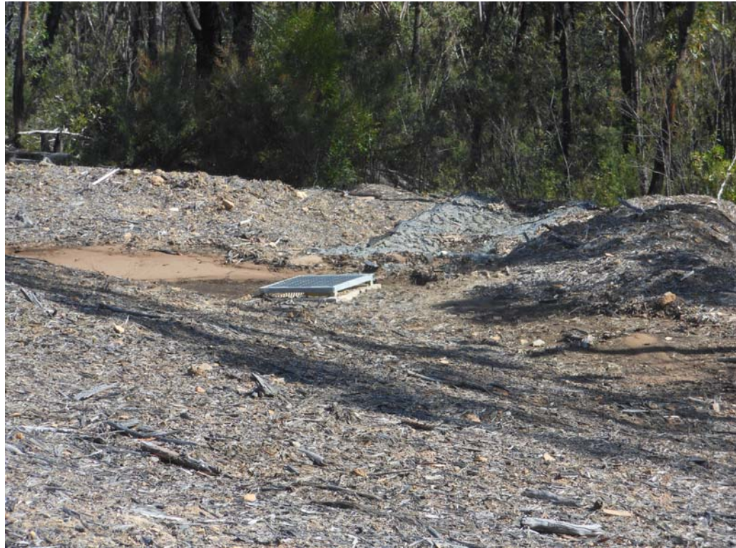
Photo 31 – Sediment drain at north-west corner of 500m Range, weed free
